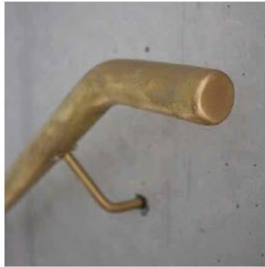
MW:01 - BRASS METAL FINISH TO BALUSTRADES
