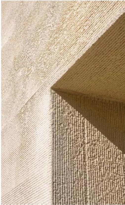
SDS:01 - GOSFORD QUARRIES WHITE TO MID SANDSTONE CLADDING - RAKED FINISH
