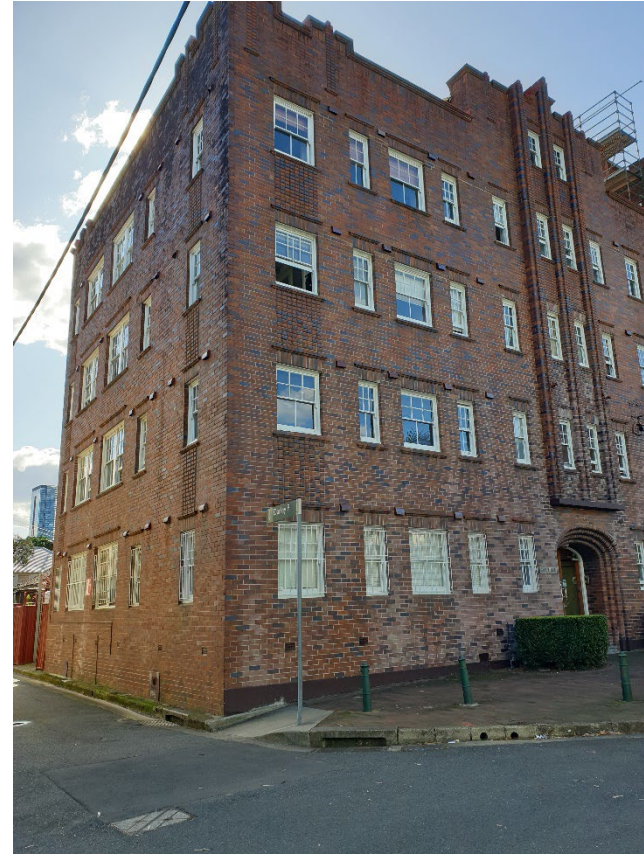
5 Darley Street to the east - viewed from Darley Street
